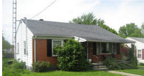
413 Bell Street – Paris – $79,500. Energy efficient two bedroom, one bath home with a detached one-car garage with an addeed open shed. Large formal living room, spacious kitchen/dining area, plus an open center hallway with pull-down stair access to the floored attic. Conveniently located, with many extras including hard wood flooring, forced air gas furnace with central air, replacement windows, and an inviting covered concrete front porch. Call today to schedule your private inspection.
