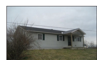
1530 Locust Grove Rd, Carlisle $39,900 Mark Mattox 289-5720 749-0828
