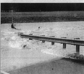
Denver Brown photo Roads were flooded in many counties after two days of rain which swelled the Licking River over its banks.
