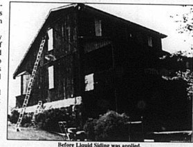
Before Liquid Siding was applied.
