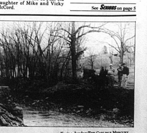
The bridge on Cranton Creek Rd. was destroyed during the flood last Friday. The damages are estimated at around $125,000.
