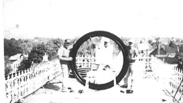
From left, General Restoration's Larry Stamer, Ed Huffine, and James Abel display a new custom made wooden ring for placement on the clock faces.
