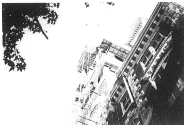
This photo shows the massive scaffolding used during renovation.
