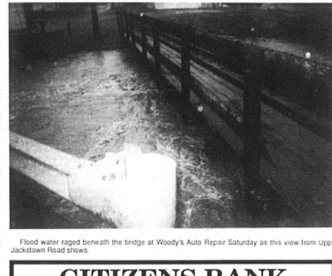
Flood water raged beneath the bridge at Woody's Auto Repair Saturday as this view from Upper Jackstown Road shows.
