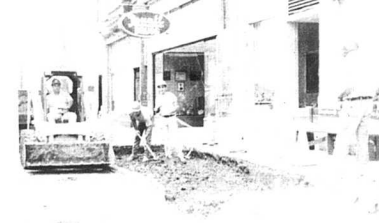
Handicap ramp installed The Nicholas County Senior Citizens Center handicap ramp was installed last Thursday. The milling lobby by area merchants. Shown are workers Wayne Smith, James Phillips, Raymond White, Bill Leforge, DOT, and foreman Jackie Hanson.
