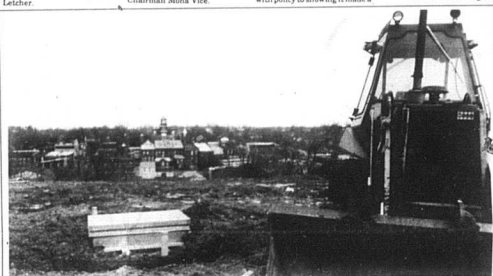
New water tower to see panoramic view of Carlisle The foundation is laid for the new water tower soon to be installed at the end of Rayne Street, said Carlisle Mayor Ronnie Clark. Contractors finished the foundation and are awaiting the steel needed to build the new tower which will provide storage of a half million gallons of water. Clark estimates the job to be completed in August.
