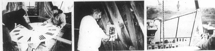
Frank Brent and Ed Huffine attach the minute and hour hands on one side of the clock face.
