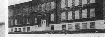
This photo taken from Ann Bow's 1952 high school yearbook shows the 'new' Nicholas County High School building in Carlisle.
