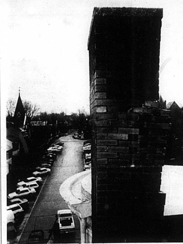
The chimney atop the Depot Bank of Carlisle began to sway this week with high winds that swept through the area Tuesday afternoon. The mortar also began crumbling and the bricks began falling.
