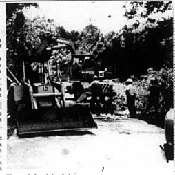
Troubled bridge This bridge or pipeline on Cassidy Creek Road is currently under repairs...
