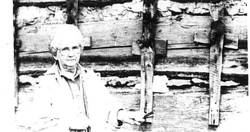
Old nails and weatherboard as they look now at the Loretta Mann residence on Highway 32 during the restoration of the 1600s home.
