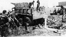
National Guard installs dry hydrant
