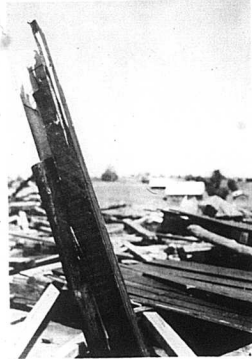
The remains of the newly remodelled six-bent barn owned by R. S. Wilts are shown here, except for what was swept away by the severe wind of the storm.
