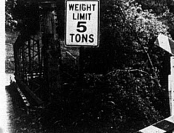
Hinkle Contracting of Paris began work on Abner's Mill Bridge two weeks ago. The old bridge, to the left, will be replaced by a new two-lane structure. The bridge being replaced is estimated to have been built in 1914.
