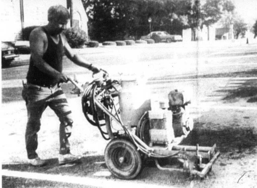
The City of Carlisle used a stripping machine to repair faded parking space lines around the Nicholas County courthouse and city building last week.
