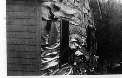
The Nicholas County Fire Department responded to a fire at the residence of James Beecraft on Upper Sharpburg Road at 1:35 p.m. last Wednesday. The owner was burning old house next to residence. The fire got out of control setting residence on fire. The fire burnt sidings and insulation on the end of the residence according to the Nicholas County Fire Chief Mark Hughes.
