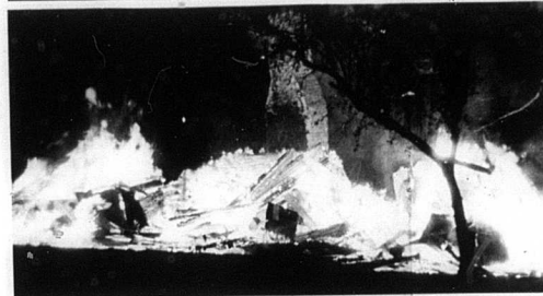
The Carlisle Mercury/Pam Bowles Photo Fire completely destroyed a home occupied by the Jerry Barnett family, owned by Junior Maxey, on Dayton Chapel Road, according to a Nicholas County Fire Department report. The structure, a total loss was completely involved upon arrival by fire fighters, Saturday night. An arson investigator was called to the scene, and the fire is still under investigation.
