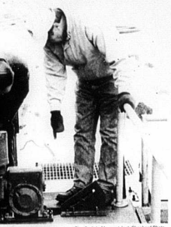
Shower plant manager Gene Kelly explains problems the missing chain on the crawler his posed the sewer plant to Carlisle Mayor Frankie Hughes.
