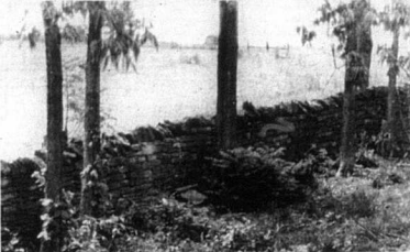
Tom Soper, a stone mason, is preserving both the art of stone work and the history of Kentucky. Soper adapts his work to conditions as seen here on this 200 feet of uphill repair work on the Shumate farm. - Heather Mathes Photo
