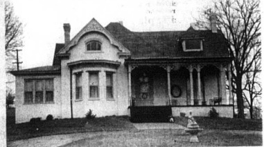
Ike and Debbie France's residence estimated to have been built during the Reconstruction period following the Civil War. After suffering much damage, the house has been almost completely restored, and reconstructed by the present owners. - Heather Mathes Photo
