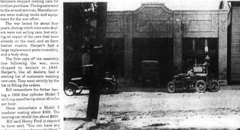
This picture shows the original Harper's Garage building before the addition was added to the right, or the parking lot was built to the left. The date of the picture has to be between 1927 when the first building was constructed, and 1928 when the second building went up. The photo belongs to Nate Young.
