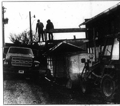
City employees worked hard to install new filters for the Carlisle City Water Plant over the Christmas holidays. Replacement of the 22-year-old filtering system began December 17, with the two-week shut-down of Jockey International. The hull in water demand made it possible for the
