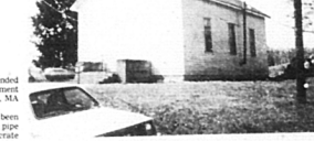
Ishmael Chapel Church The Ishmael Chapel Church, located on Ishmael Road, has had a location discovered in the 'before' 'top' and 'after' (bottom) photos. Work is still being done on the inside by church members. According to Carl Ishmael, the church was built in 1874 by Mr. Ishmael's grandfather, Timothy Ishmael, his great-grandfather, Samuel Ishmael, who deeded the land to the church, and church members. The present pastor is Alvin E. Kiser, who ministers to 25 members.
