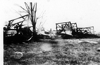
13 bent barn destroyed
