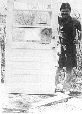
Forced entry Don Short, manager of the Dairy Queen, is pictured holding the back door of the building that someone tried to break down last Tuesday night. April 1 in a robbery attempt. A metal door is being installed in its place.
