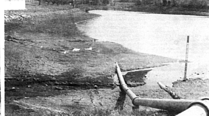
Dry bed, almost The water level of the city lake was lowered four or five feet last week in order to prevent possible flooding through a hole that was discovered in the dam. A suction pipe, visible in the foreground, was one of several used to lower the water level. This shot was taken Sunday afternoon. —Guthrie Photo
