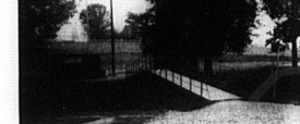
New footbridge to park A new footbridge leading to the East End Recreation Park has been completed... just in time for Sunday's 1:30 p.m. charity horse show benefiting the Delta Livestock and Feeds Howden fund. The spot with constructed with matching funds from a recent federal grant to improve park facilities. —Mercury photo
