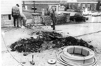
Gas line work almost finished
