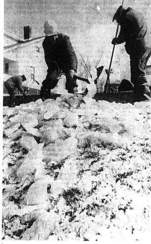
City of Carlisle employees work last week to chip some accumulated ice from a curve on the Upper Jackstown Road at the city limits. Drainage from private residences gathers so the men and freezes in cold weather. The men are, from left, Bill Mitchell, Cleo Fryman and Vernon Willschlagby. — Photo by Jeff Kerr.
