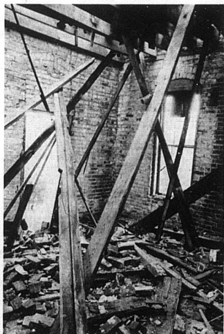
This shattered room once beamed with activity.
