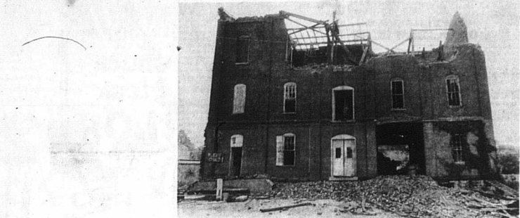
The mill as demolition progresses.
