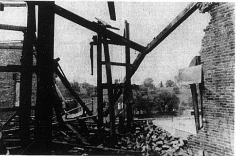
The third story is now roofless.
