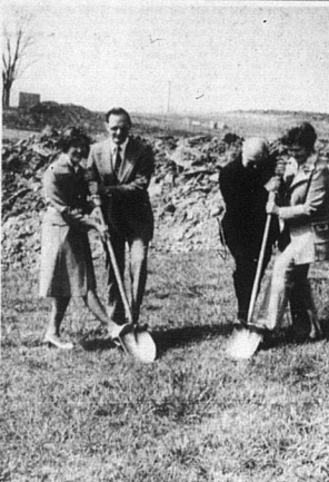
New hospital site
