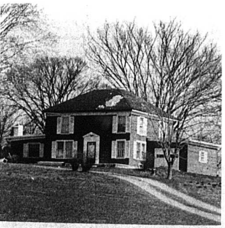
Garrett Gray's house at Pleasant Valley was meted extensive damages. The front porch was torn off, blown over the house, and set down in the back yard of the house. The columns to the porch were left in front. The spot where one of the three destroyed chimneys was located can be seen on the roof.—Mercury photo
