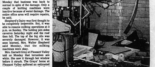
Water damage was extensive at Blue Grass Knitting as the sprinkler system was activated. After clean-up operations during the weekend business was conducted as usual on Monday morning except for the office area. Only two knitting machines remained inoperable Monday.—Mercury photo
