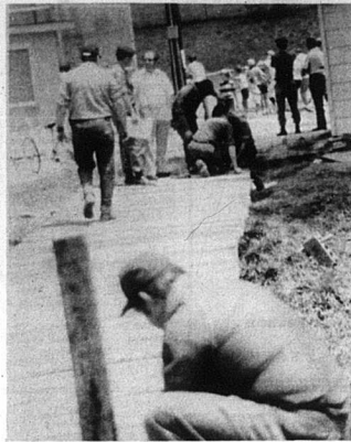
Recreation Park gets new bridge; bleacher repairs
