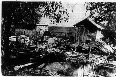
Headquarters Road home destroyed
