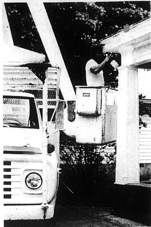
It's much easier and safer to use a "cherry picker" to get a painting job done... that is if one is available. Danny Boone, a construction worker, is
