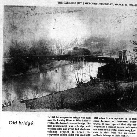
In 1836 this suspension bridge was built upon the Licking River at Blue Licks. In 1917 when it was replaced by an iron span because of increased heavy traffic, it was reported that only one wagon and a team of horses could cross side at a time as the bridge would sway from side to side from the movement. Photo belongs to Bob Fisher.
