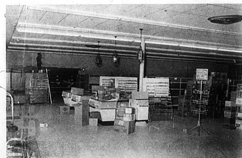
Near ceiling in the upper left is Paul Stone, Kentucky Utilities employee, who with the help of Samuel E. Wilson did the electrical wiring in the store.
