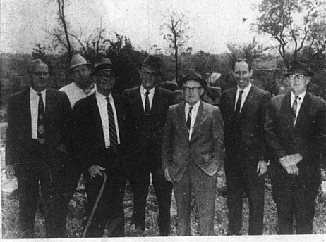
Six members of the First Christian Church and their minister, Rev. Neil Thompson, braved wet grass and Nicholas County clay Sunday afternoon to pose for the Mercury photographer at the scene of earth moving for the foundation of their new church building.
