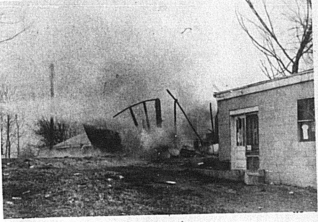
PLENTY OF WATER IS SHOOTING ACROSS THIS BLAZE.—That is thought to have resulted from a defective line in the front part of the building. An alarm turned in at approximately 2 p.m. Tuesday was answered by both City and County fire units, the City truck going to the McCarty home where a fire was being fought. A house to the right of the fire in the left part of the picture got under control from the McCarty home. Fire Chief Woodrow Wilson stated he answered his fire phone but was unable to sound an alarm due to a malfunction of the strage system. He added he called the Police station in an attempt to have them report the fire, but no one was there. Finally the alarm blaze was fed by oil from a 150 gallon tank, the edge of which had blown above the County unit returned to the scene to assist a fire reported as a City fire drill.—Mercury photo
