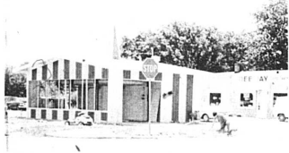
FINISHING TOUCHES are being made to the grounds by Dennis Hunt as his father, Clay Hunt and William Duncan do the mechanical work on the inside of this automatic car washer which will be put into operation soon.
