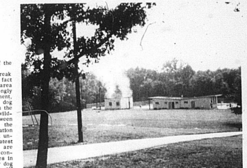
IN A CLOUD OF CHLORINE GAS—This view of the Blue Licks State Park pool pump house was taken by Johnny White, Nicholas County Sunlight Club, Monday, August 5. The black object near the building slightly in the foreground is one of the chlorine gas tanks that was blown through the roof of the building.
