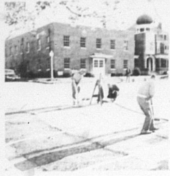
MARKING PARKING SPACES—Brooks Henson and a crew of city workers mark parking area in front of the Carlisle Christian Church. Marking or painting a stripe is being done with a special brush purchased by the city for this purpose. With well marked areas there is little excuse for improper parking.—Mercury photo.
