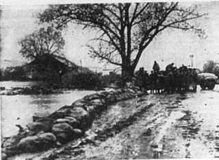
DONATEE CAPES and Fred Perrenot are shown after strengthening a levee near Great Falls, Mont., which in the past is a record flood on the River. Strongly flooded areas around the river to west which in the past is a record flood on the River. Strongly flooded areas around the river to west which in the past is a record flood on the River. Strongly flooded areas around the river to west which in the past is a record flood on the River.
