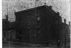
NICHOLAS COUNTY JAIL This picture shows the Nicholas County Jail in 1900. It had been remodelled in 1892.
