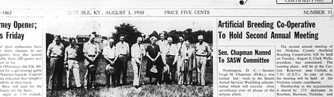
GROUND BREAKING CEREMONIES FOR THE NEW NICHOLAS COUNTY HIGH SCHOOL...
