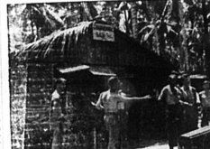
Telephone Exchange on Guadalcanal
